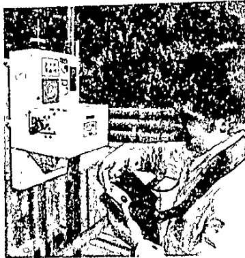
△ Taking a reading from a static air sampler in the Fuel Handling Plant.
